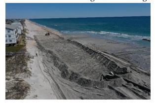
on the beach just south of Queens Grant. This is where the initial placement of sand will begin and move north to the town limits. Once completed, the pipeline will be flipped, and the process will move south towards the Jolly Roger Pier. In the meantime, Weeks Marine continues to prepare for the arrival of the second dredge, the *Boringuen*. Once here, the *Boringuen* will
